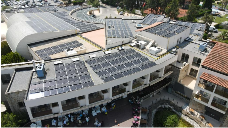
Solar panels and Electric panels
